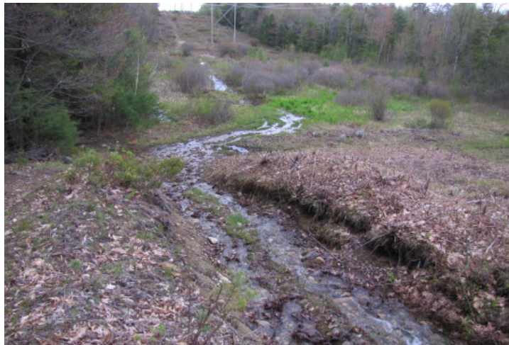
The powerline access road is severely eroded above Wetland G; fortunately, this wetland is exceptional at Nutrient Transformation
